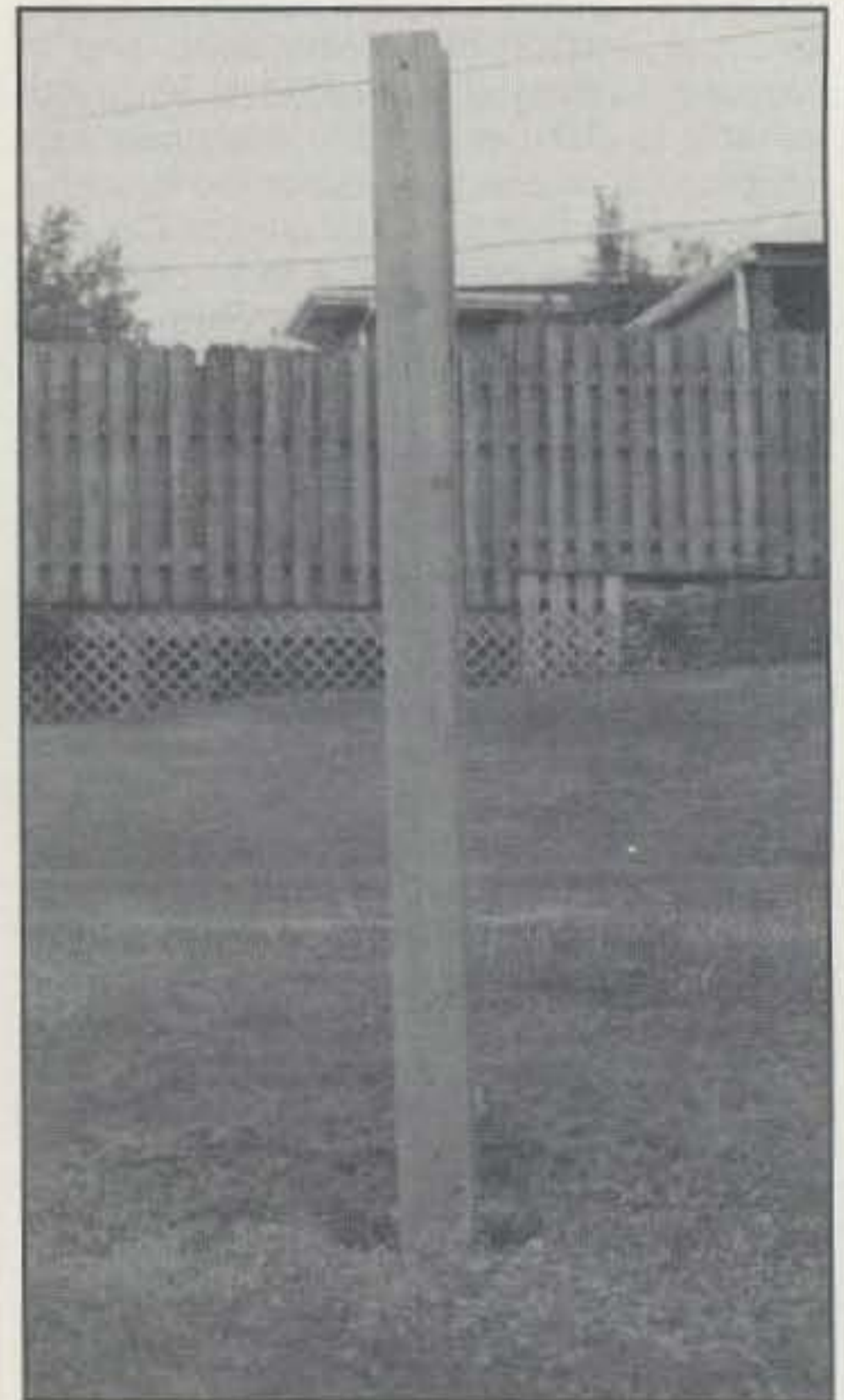
Be sure the wooden supports are vertical and plumb.
